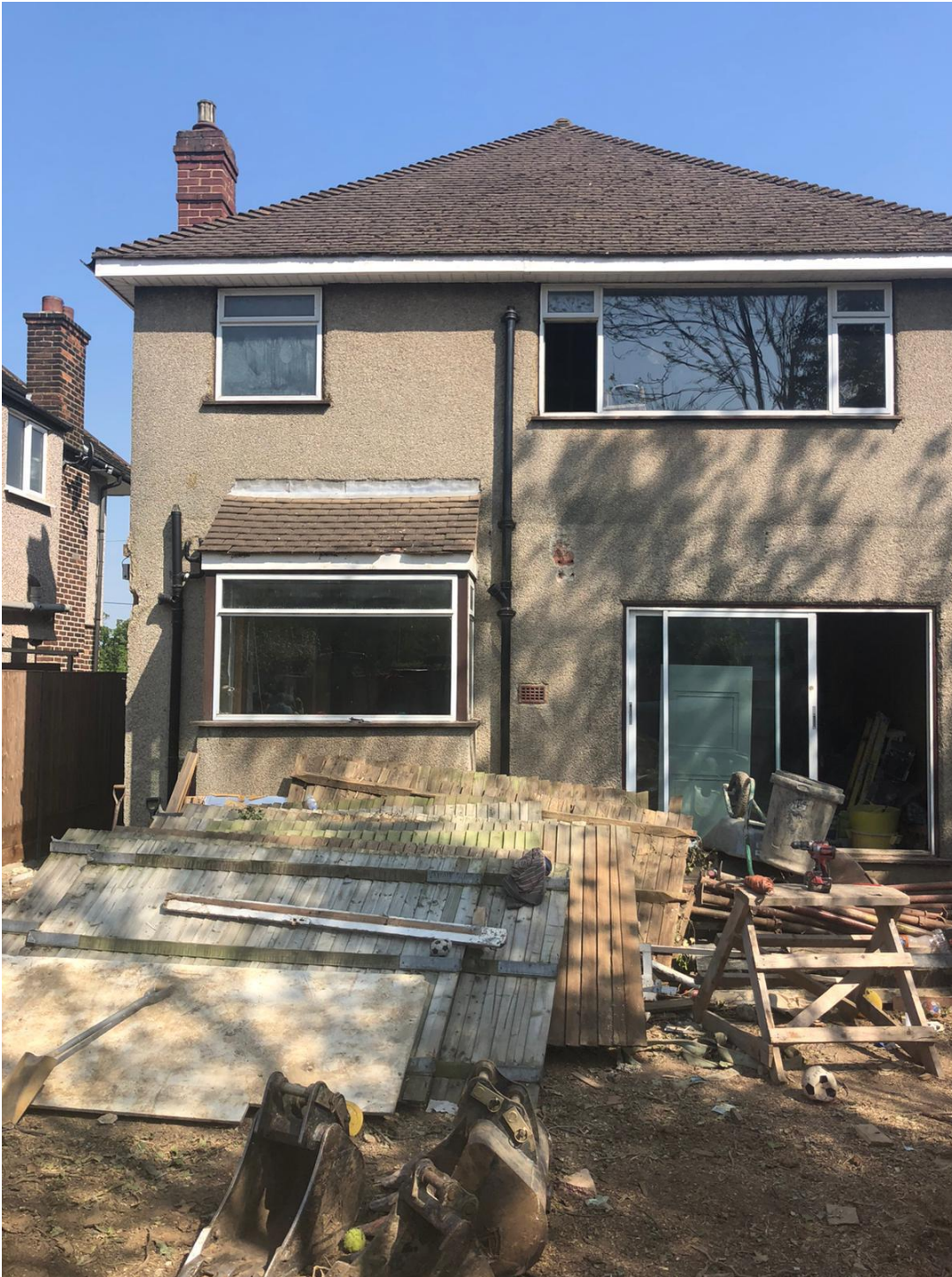
Figure 2 – Existing rear elevation of subject dwelling
